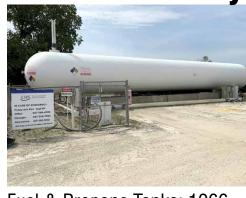
Fuel & Propane Tanks: 1966 Cherokee 30,000 Gallon Propane Storage Tank Fuel Station with Overhead Fill, 1 Pump with Electric Motor & Veeder-Root Meter
